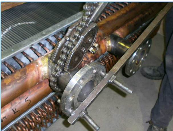
Installing screw-on flange
