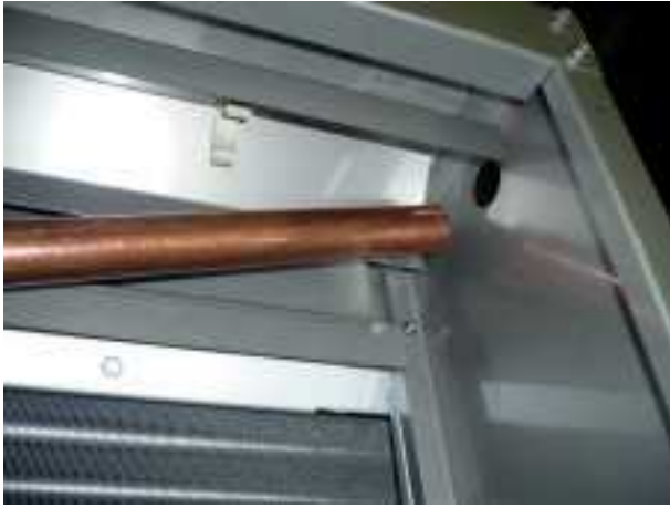
Installation of copper waterfeed pipe
