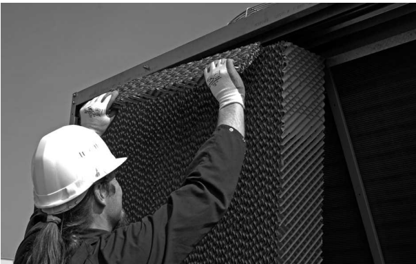
Removal water distribution pads
