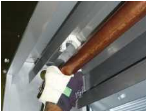
Release copper collector from plastic holders
