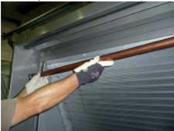
Remove copper waterfeed pipe
