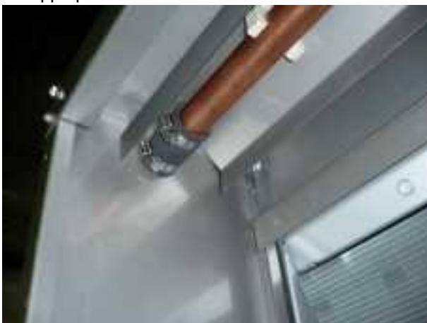
Flexible sleeve connection
