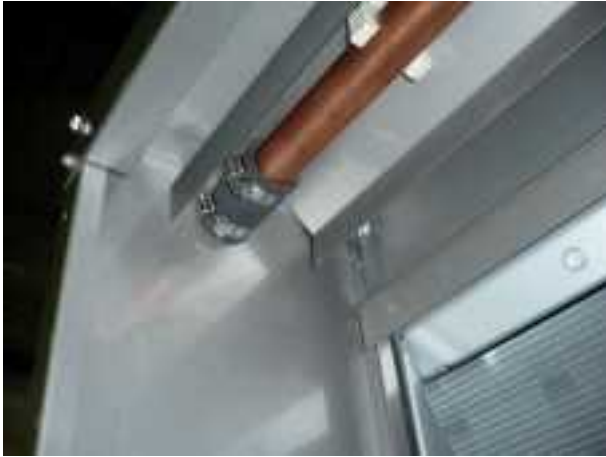
Flexible sleeve connection with sleeve clamps
