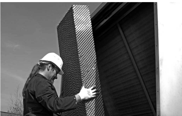
Removal pre-cooling media
