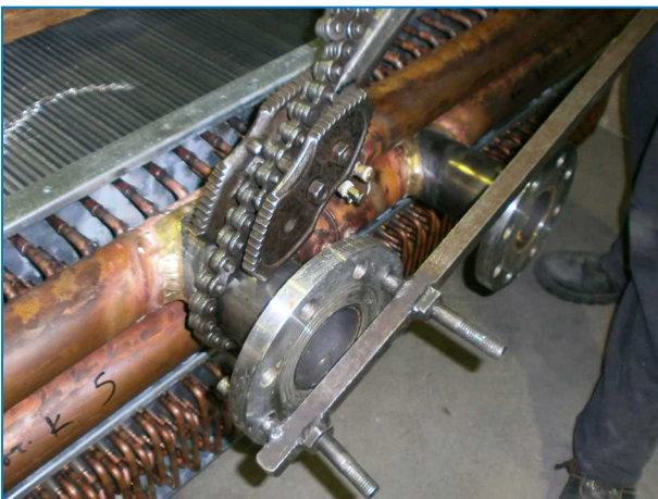
Installing screw-on flange
