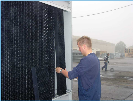
Remove combined inlet shields
