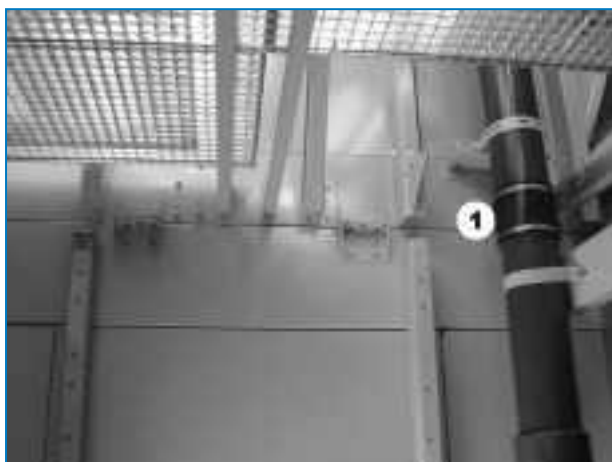
Sleeve with hose clamps
