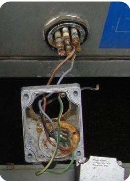
The heater is burst and deformed due to overheating. Once the element is open by bursting, water will enter and flow to the connection box, starting corrosion and short circuiting.
