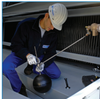
on site services
