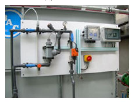
BAC offers a wide range of **automatic water treatment packages** to control corrosion, scaling, fouling and microbiological growth in cooling systems incorporating BAC cooling towers.
