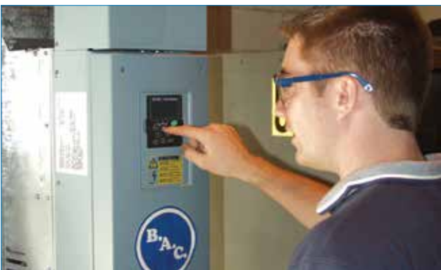
Figure 8: VFD with Integrated Bypass
