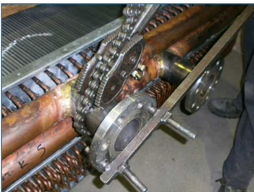
Installing screw-on flange
