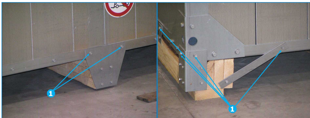
Removal of shipping skids – Side view & End view
