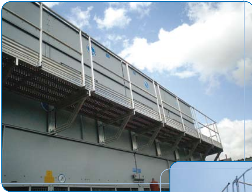
BAC Model VXI Closed Circuit Cooling Tower with Discharge Sound Attenuation Package
