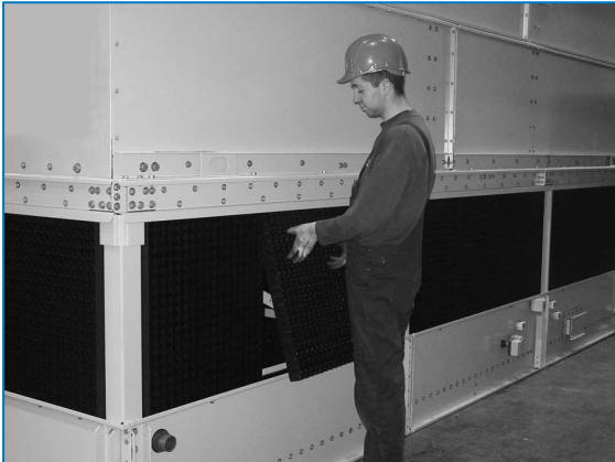
Remove combined inlet shields
