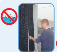
Protection of spray water from sun, debris and avoids water splash out during fan cycling
