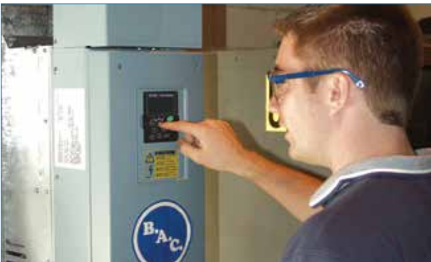
Figure 8: VFD with Integrated Bypass
