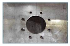
Flat Face Flange pattern is shown on this cold water basin panel to suit a EN 1092 flange
