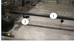
Figure 4: Sump Sweeper Piping 1. Pressure Pipe; 2. Eductor.
