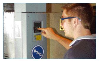
Figure 8: VFD with Integrated Bypass
