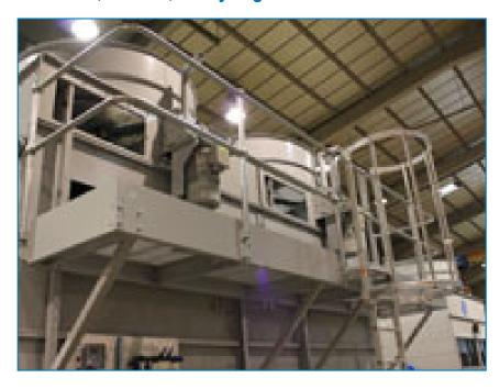
**Platforms**, a ladder, safety cage and handrails facilitate easier and safer access to the top level of the unit, making inspection and maintenance easier and conforming to European safety standards.
