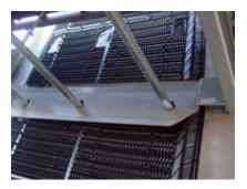
The patented VersaCross fill is designed and tested in the <u>BAC</u> <u>laboratories</u>.
